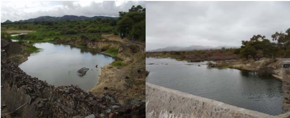
Zipwa Dam during and after reconstruction
